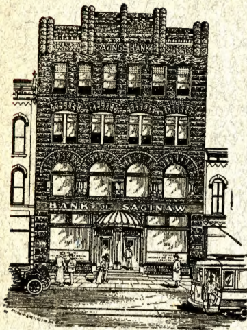
EAST SIDE OFFICE, #10-112 GENESEE AVENUE.
